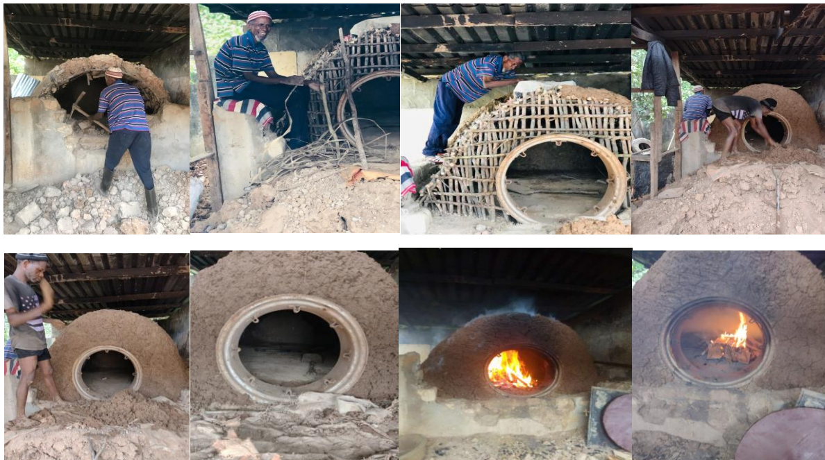
Figure 1: Photos taken from the construction site
